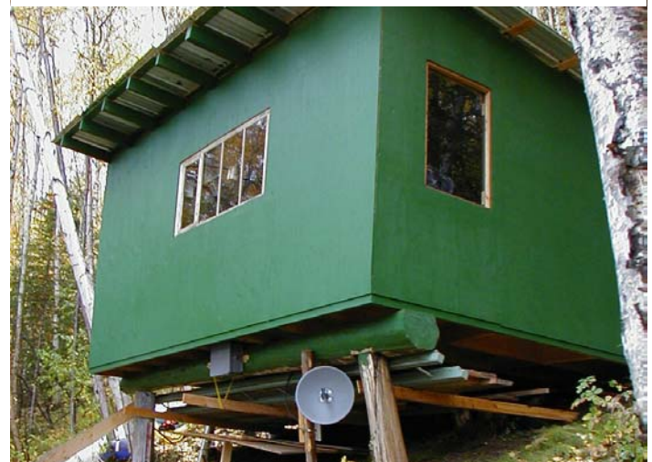
Rapids video shack with microwave dish for receiving video for computer fish counting.
