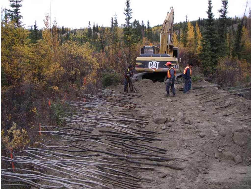
Photo 6. Willow and poplar stakes incorporated into the berm (brush layers).
