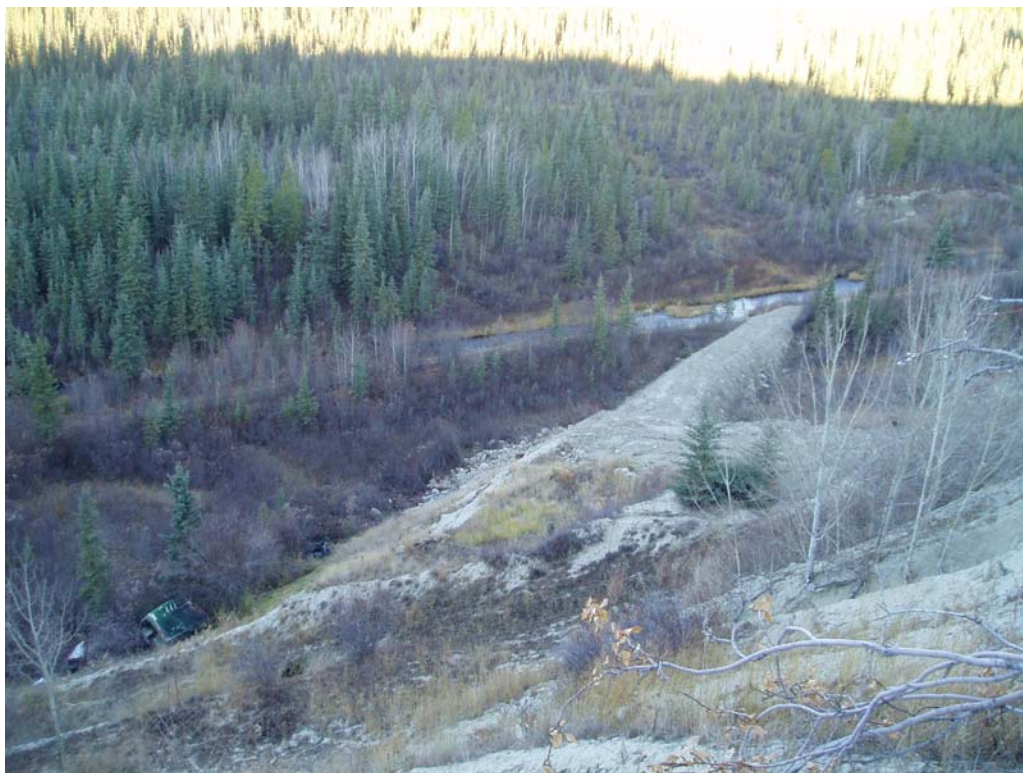
Photo 8. Completed berm with McIntyre Creek in background (flowing left to right).
