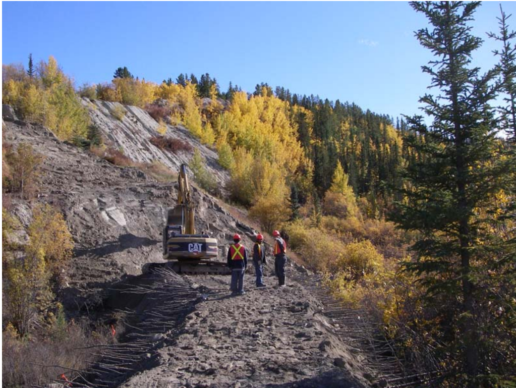
Photo 7. Berm nearing completion, taken from old berm location near McIntyre Creek.
