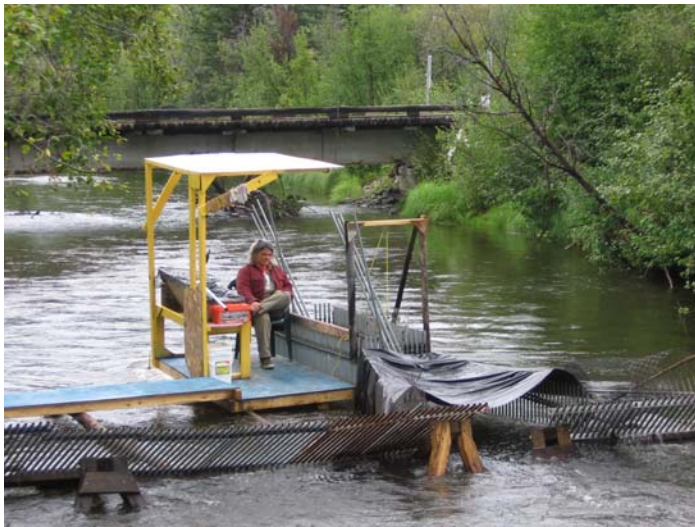
Figure 2. View of counting chamber and sampling station looking upstream.
